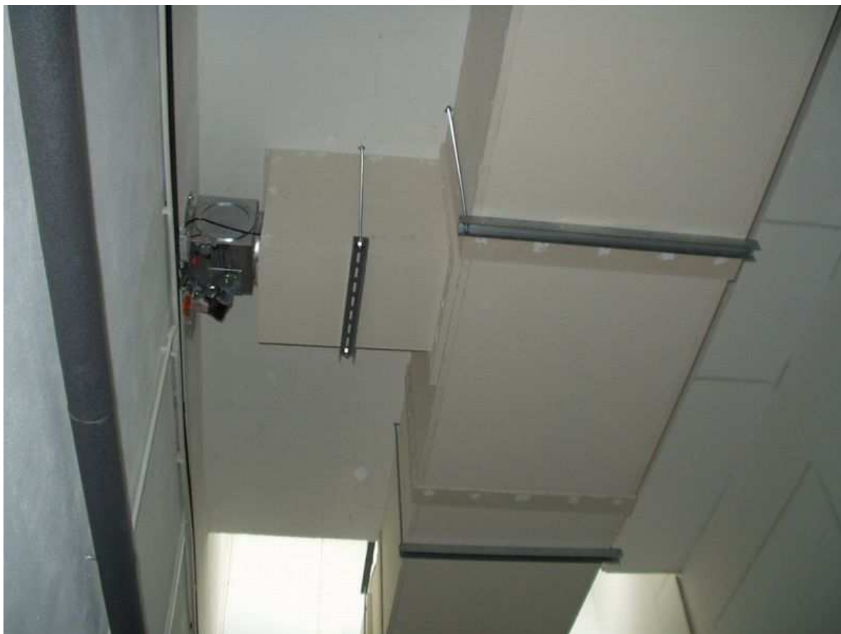
Obr. 4 Izolácia VZT potrubia. Tunel Branisko Fig. 4 Air duct insulation. Tunnel Branisko
