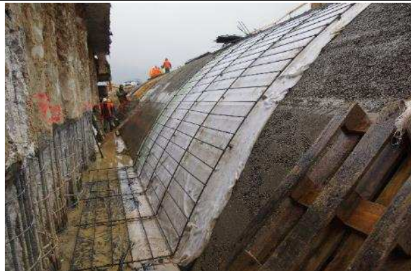
Obr. 9 Separáčn  vrstvy a mont z v ztu e  elvy Fig. 9 Separation layers and the placement of the “tortoise shell” concrete reinforcement
