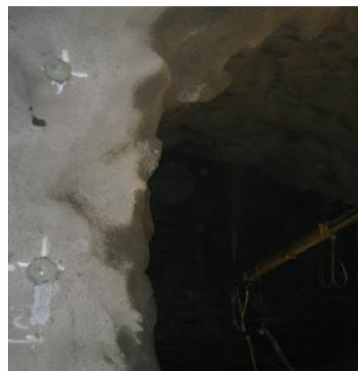
Shotcreting in the Götatunnel
