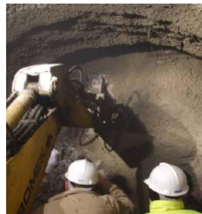
Tunnel excavation by crusher
