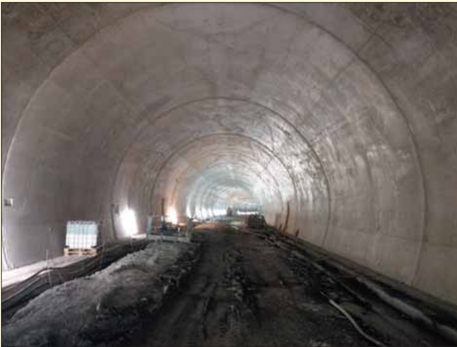
Obr. 7 Sekundárne ostenie tunela Milochovo Fig. 7 Secondary lining of the Milochovo tunnel
