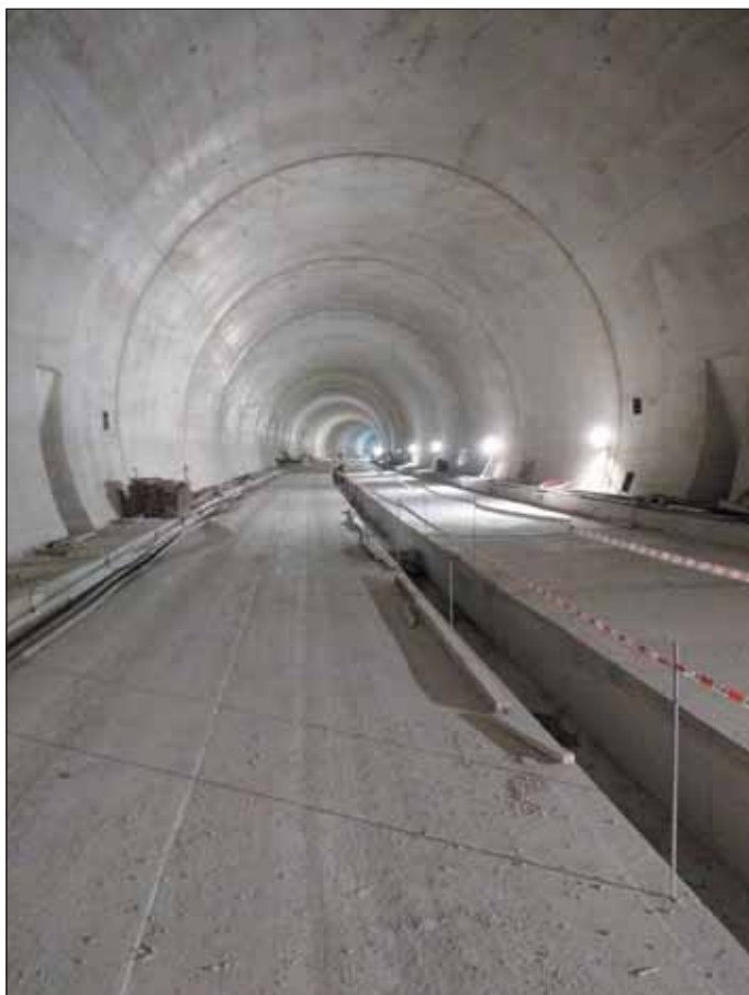
Obr. 1 Sekundárne ostenie tunela Diel Fig. 1 Secondary lining of the Diel tunnel
