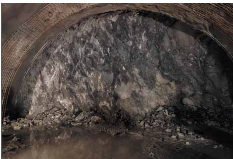
Obr. 2 Razenie tunelu Milochovo Fig. 2 Excavation of the Milochovo tunnel
