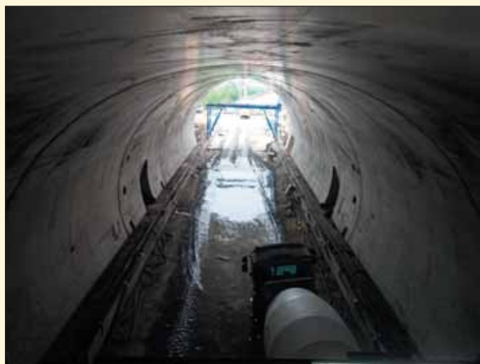
Obr. 8 Tunel Diel – sekundárne ostenie Fig. 8 Diel tunnel – secondary lining
