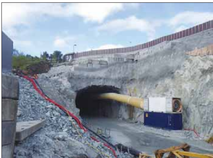
Obr. 7 Tunel Solhei Fig. 7 Solhei Tunnel
