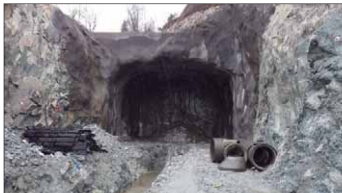
Obr. 6 Tunel Steinsvik Fig. 6 Steinsvik Tunnel
