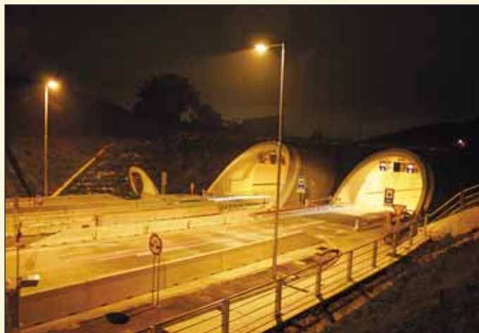
Obr. 3 Tunel Sitina – pohled na portály Obr. 3 The Sitina tunnel – view of the portal
