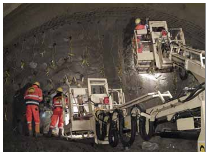
Obr. 3 Instalace elektronických rozbušek do čelby Fig. 3 Installation of electronic detonators into the excavation face
