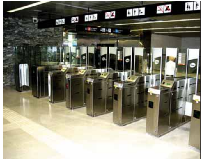
Obr. 9 Uzavřený odbavovací systém (turnikety) Fig. 9 The closed entry system (wicket gates)
