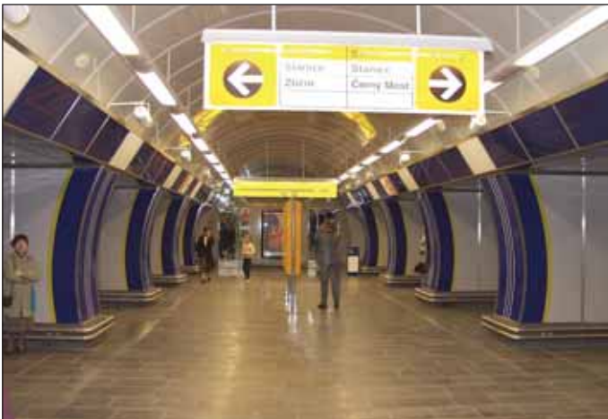
Obr. 3 Trojlodní stanice metra Kolbenova, 1990 Fig. 3 Kolbenova three-vault metro station, 1990
