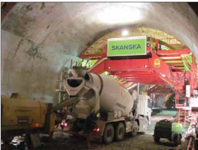
Obr. 9 Betonáž hornej klenby tunela Fig. 9 Casting of the tunnel upper vault
