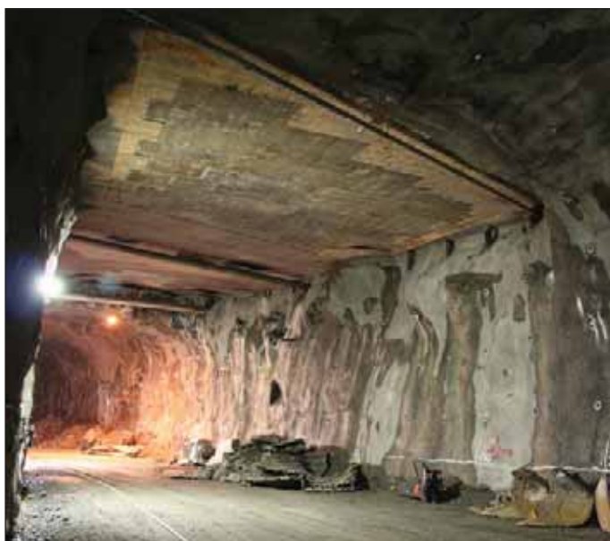
Obr. 3 Pohľad na ŽB dosku deliacu tunel 111 od tunela Eugenia Fig. 3 View of the RC slab separating tunnel 111 from Eugenia tunnel
