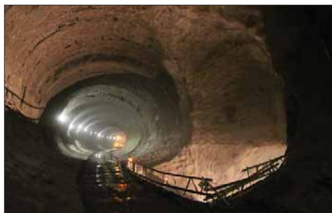
Obr. 6 Pohled z STT do spojovacího kanálu 4 Fig. 6 A view from the NTT down the connecting duct No. 4
