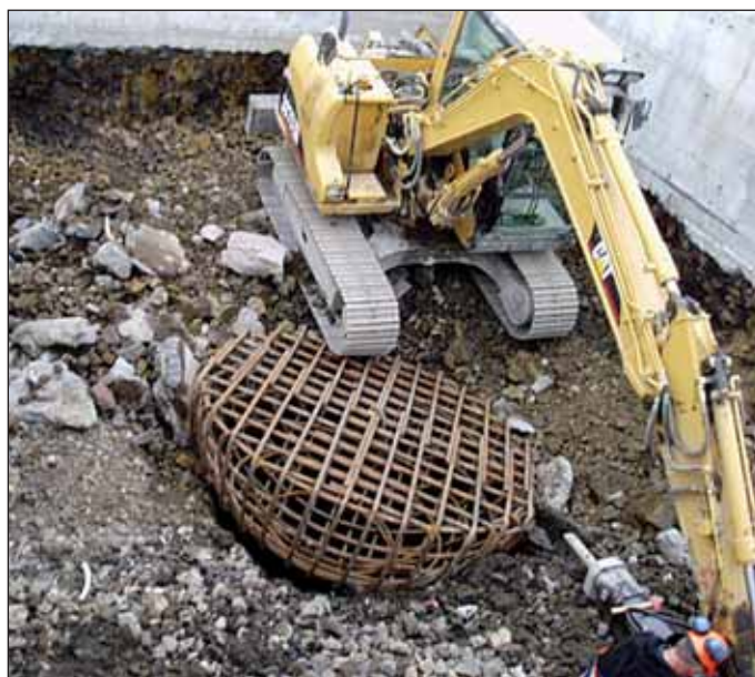
Obr. 4 Šachta pre hradidlové vráta – odtážba do predvrtu Fig. 4 The power intake gate shaft – muck removal through the pre-drilled borehole
