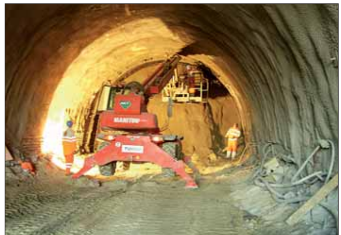
Obr. 5 Vystužovanie ostenia tunela sieťovinou Fig. 5 Reinforcing of the tunnel lining with steel mesh
