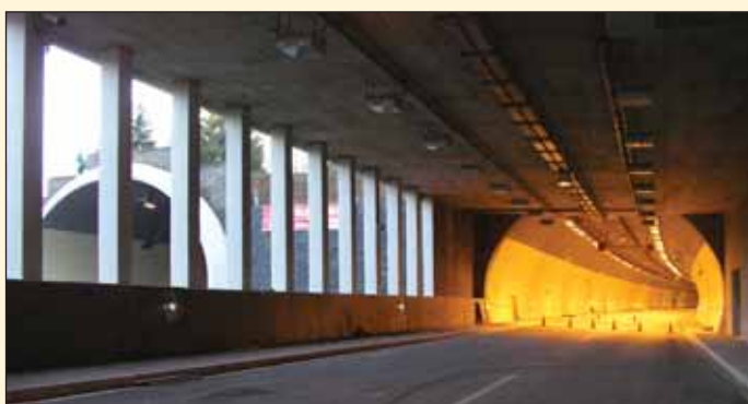
Obr. 3 Galerie u severního portálu tunelu Libouchec Fig. 3 The gallery at the northern portal of the Libouchec tunnel
