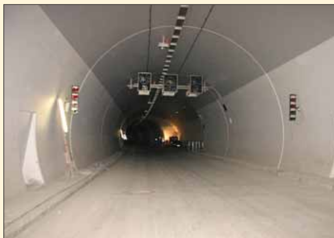
Obr. 2 Pohled do tunelu Sitina Fig. 2 View inside the Sitina tunnel
