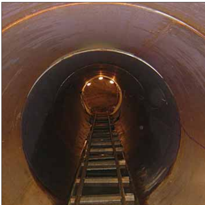
Obr. 2 Ocelová chránička a čelo protlaku Fig. 2 The steel casing pipe and front end of the pipe jack
