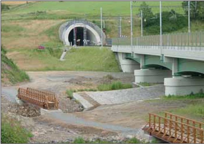
Obr. 1 Krasíkovský tunel Fig. 1 The Krasikov tunnel
