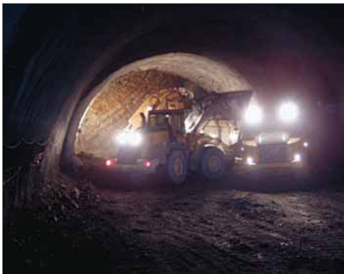
Obr. 5 Ražba kaloty STT Fig. 5 NTT top heading from the east
