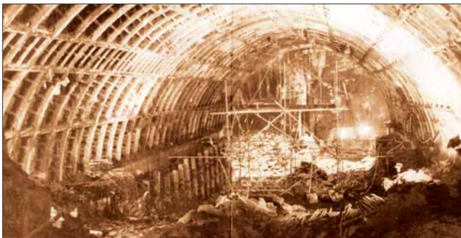
Obr. 9 Vinohradské tunely Fig. 9 The Vinohrady tunnels
