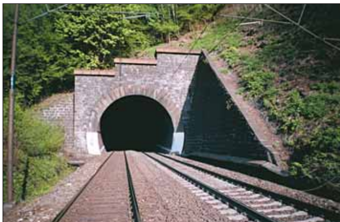
Obr. 5 Bujanovský tunel Fig. 5 The Bujanov Tunnel
