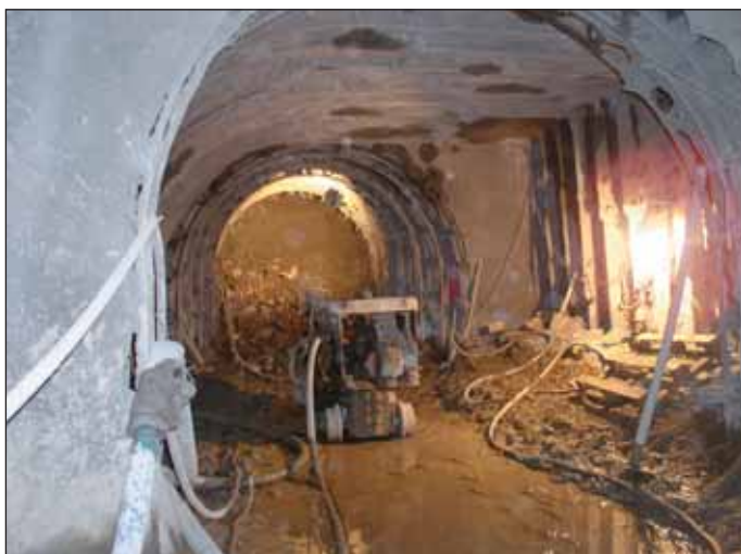
Obr. 4 Pohled na komoru K7 Fig. 4 View of the chamber K7
