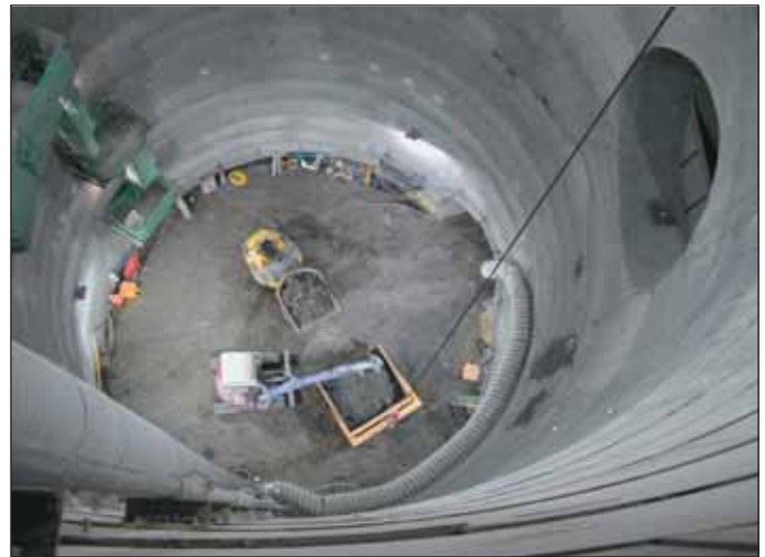
Obr. 9 Šachta T5C PiccEx Fig. 9 T5C PiccEx shaft
