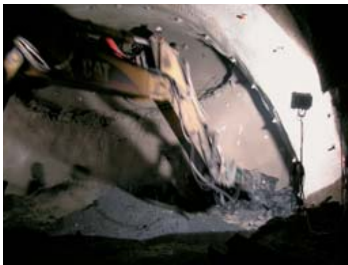
Obr. 1 Hydraulické rýpadlo CAT 330 a 320 s impaktorom Fig. 1 Hydraulic excavator CAT 330 and 320 with impactor
