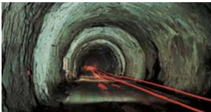
Obr. 2 Průjezd tunelem Homer Fig. 2 Passage through the Homer tunnel
